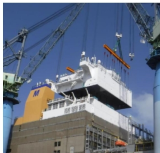
House top installation on Lurline , April 2019.
